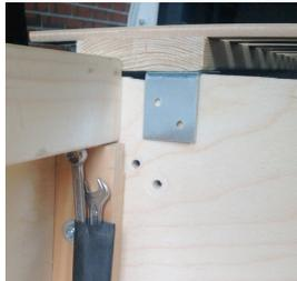
slats a bolt fits into a hole in the board, making it easy to remove. In the middle of the 3 boards I put a hinge so it can be folded for storage. An angle bracket keeps the right and left board in place. Here you see where I keep the necessary tools to put the pieces together or take them apart.
