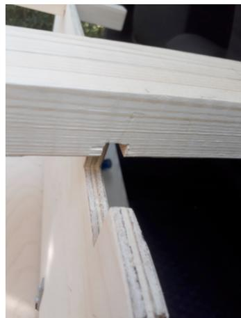
The middle lath is fastened to an alternative piece of board with bolts – and with a piece of wood between the board and the lath to give the correct height.
